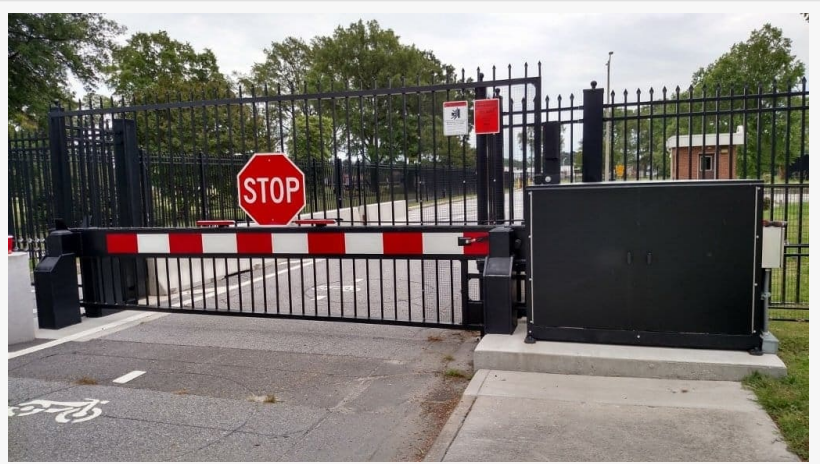
Electric Gate Repair
