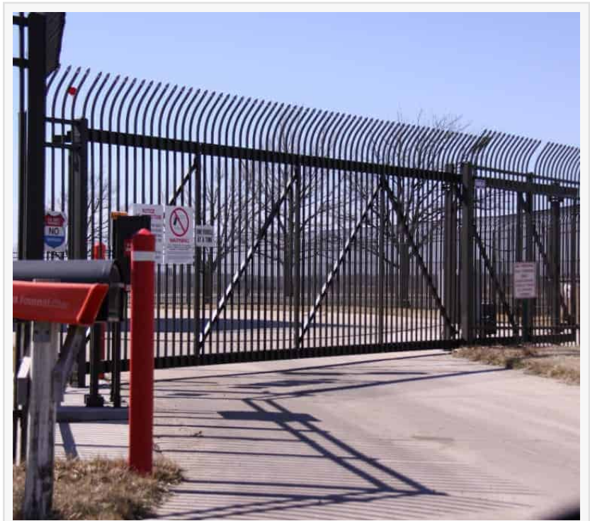
Automatic Gate Repair
