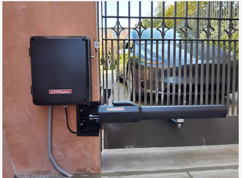
Affordable Fence Installation
