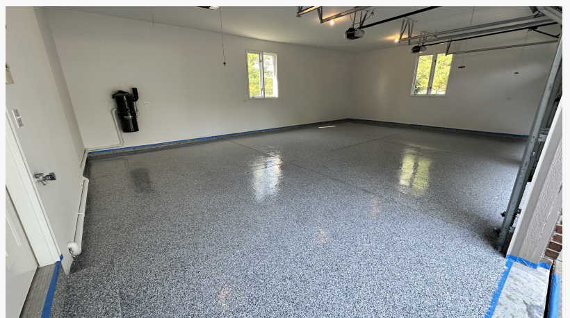
garage floor epoxy coat
