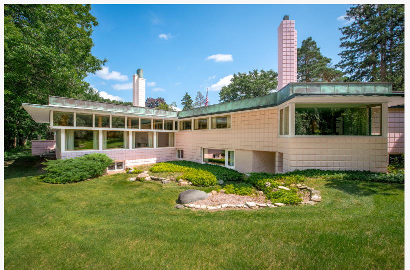
Arbury Residence Midland Michigan
