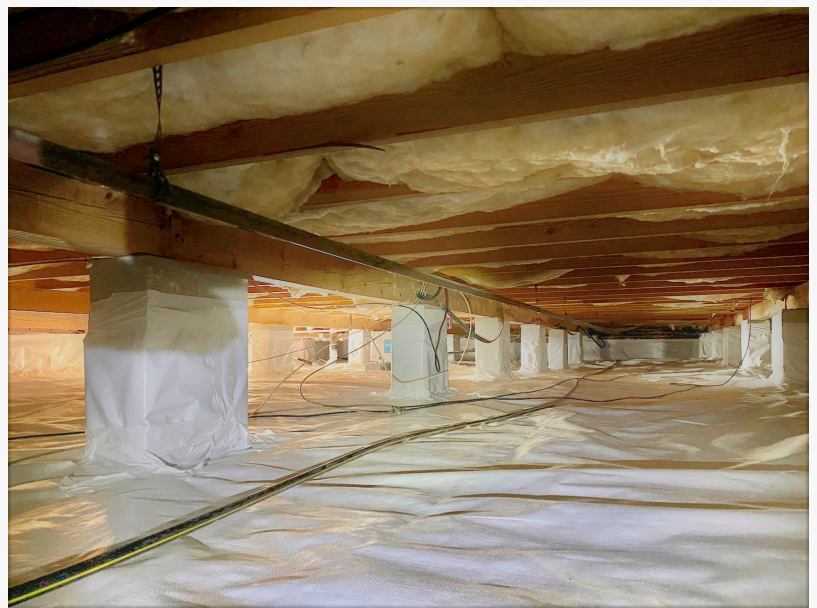
Encapsulation Under Home in Crawl Space
