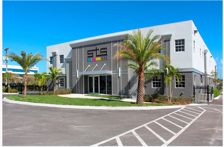
STS Inks Headquarters in Boca Raton, Florida
