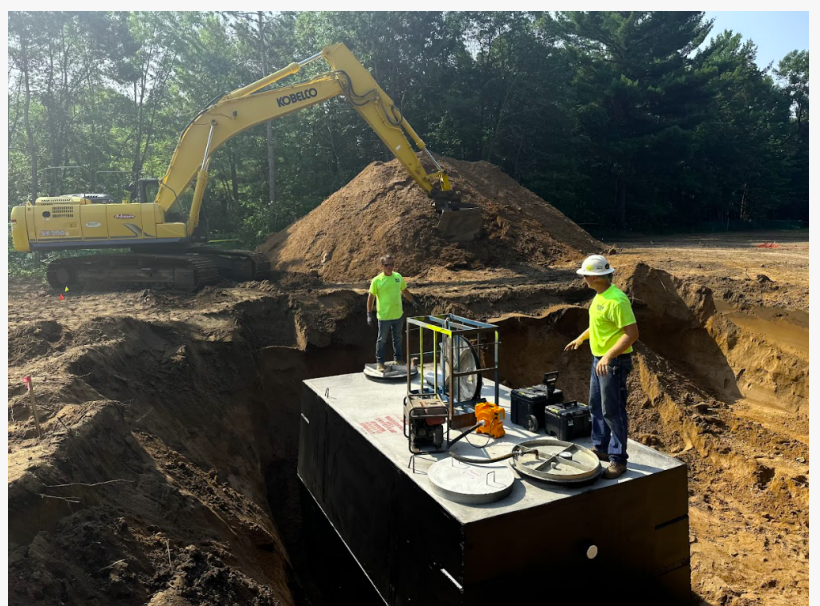
Ace Contractor Employees Hard at Work
