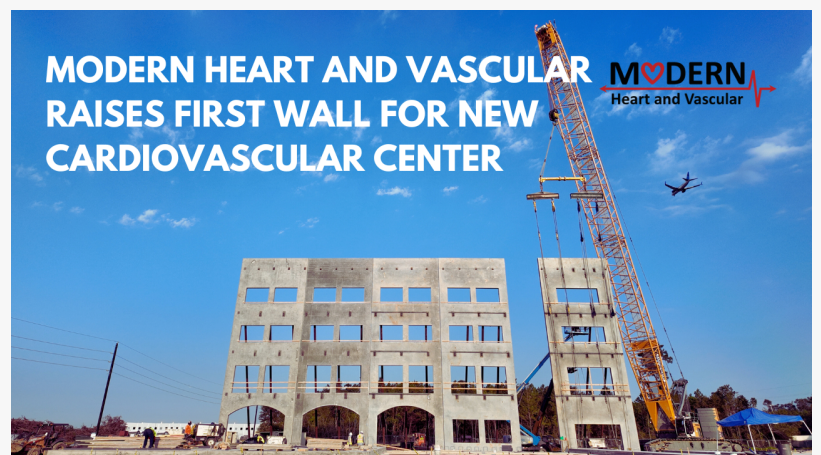
Modern Heart and Vascular Raises First Wall for their New Building
