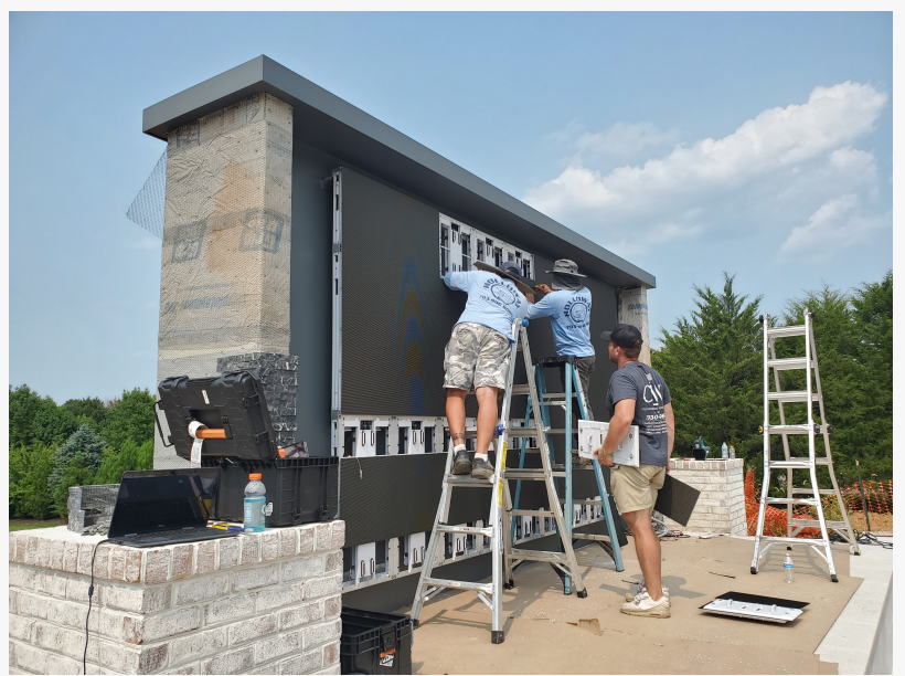
YOLO TV Partner Installation of a wall mount 202 inch Outdoor TV
