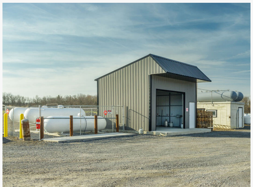
Commercial Structure Built by TriState Barn Builders
