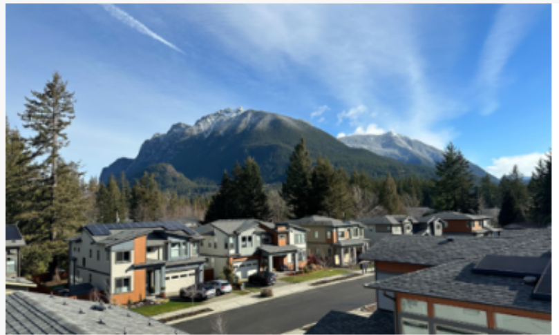
Sunergy Systems Solar Installation
