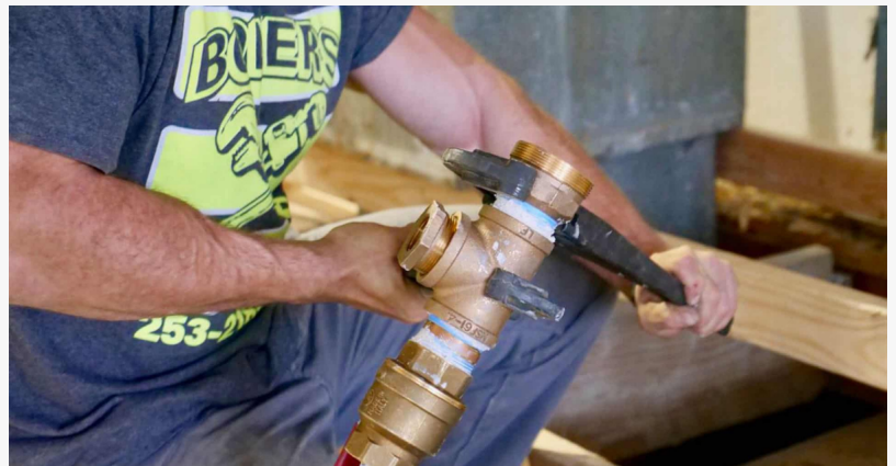
A member of the Bowers Plumbing & Remodel team at work.
