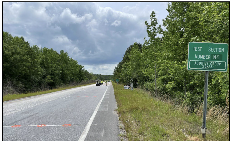
Figure 8. NCAT Test Track Section N-5 with ACE XP Aramid Fiber
