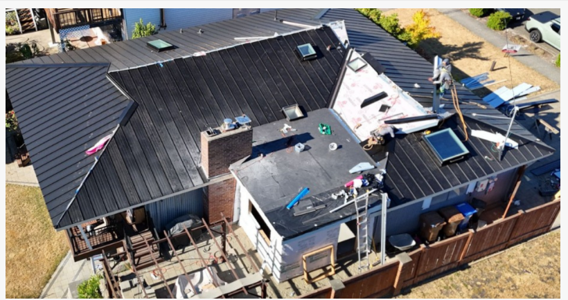
RoofSmart crew members installing a new metal roof.
