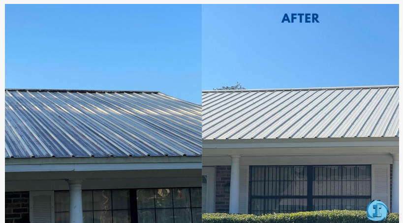
Fall Soft Wash Roof Cleaning
