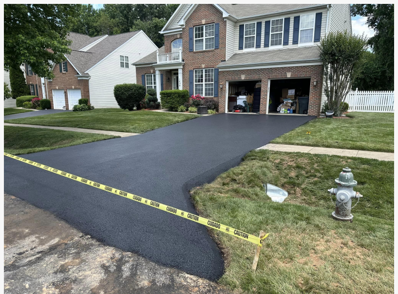
Asphalt driveway paving installation in Gaithersburg, MD
