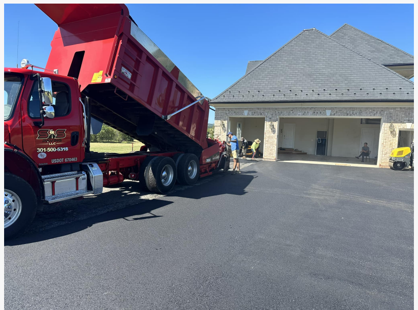
Asphalt driveway paving installation in Frederick, MD
