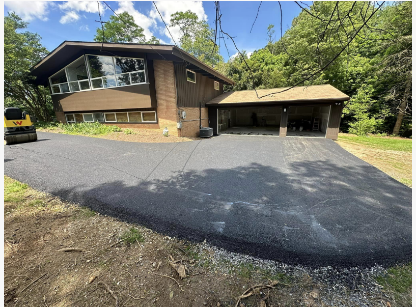
Asphalt driveway paving installation in Rockville, MD
