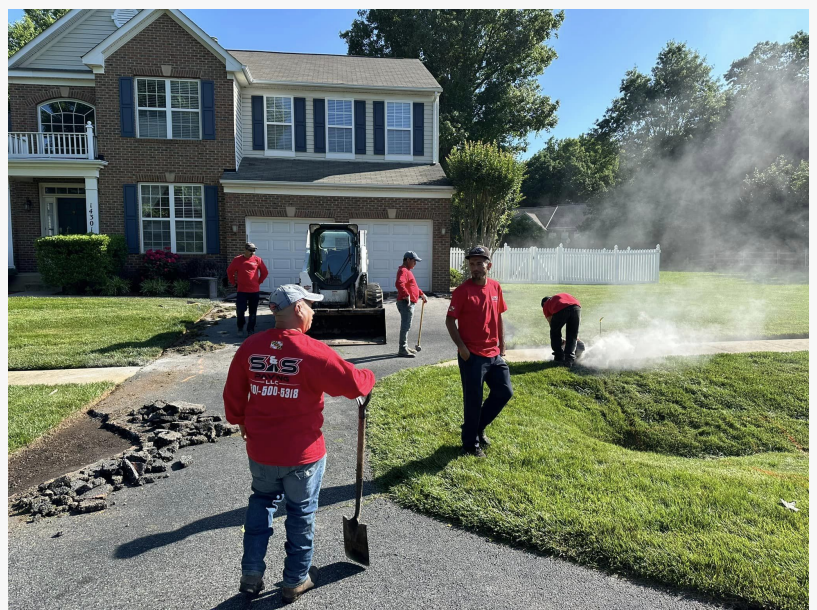
Asphalt driveway paving installation in Silver Spring, MD
