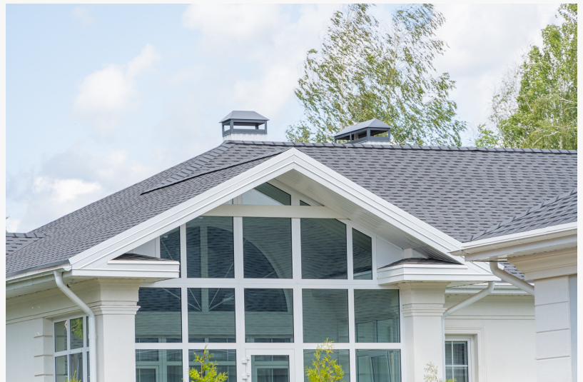
Roofing in Fort Miami, FL
