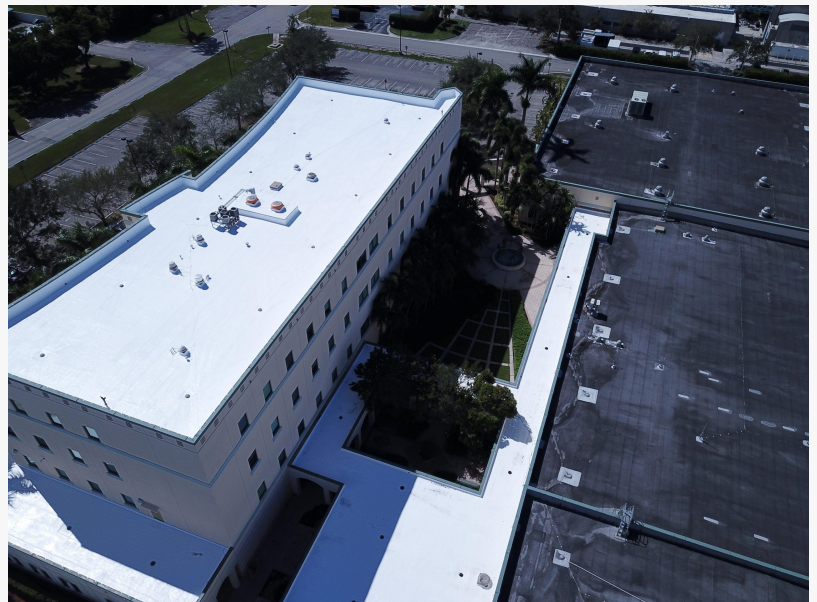
Roofing in Hialeah, FL
