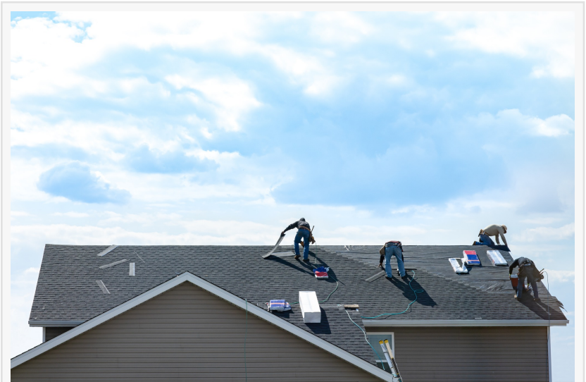
Roofing in Fort Lauderdale, FL
