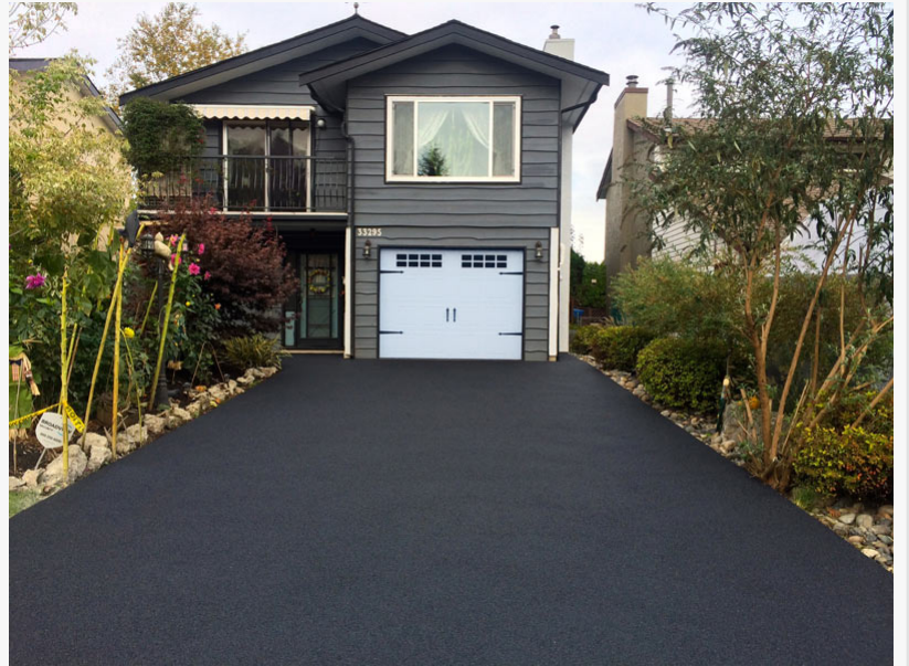
Driveway Installation in Charlotte, NC and Surrounding Areas
