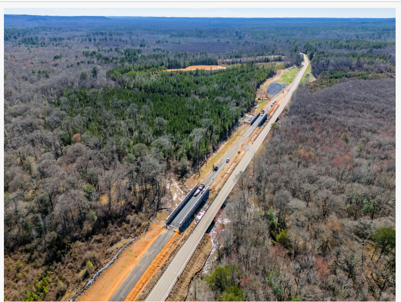
Acrow Detour Bridges in Alabama
