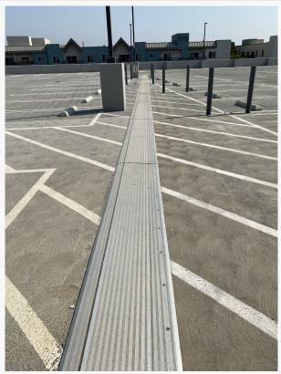
The DuraSpan portfolio consists of 16 expansion joint systems across three main categories: metal cover systems, elastomeric seal systems, and foam seal systems.
