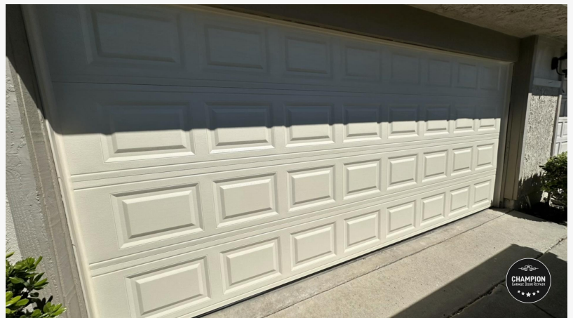
Garage Door Repair Newport Beach - After
