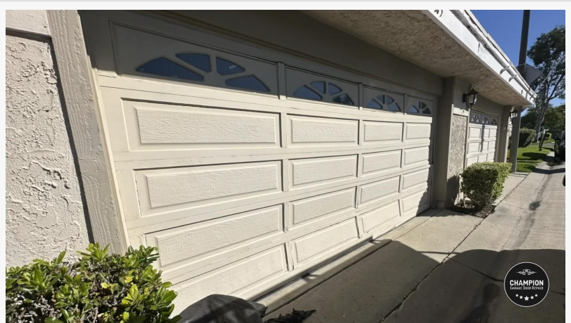
Garage Door Repair Newport Beach - Before
