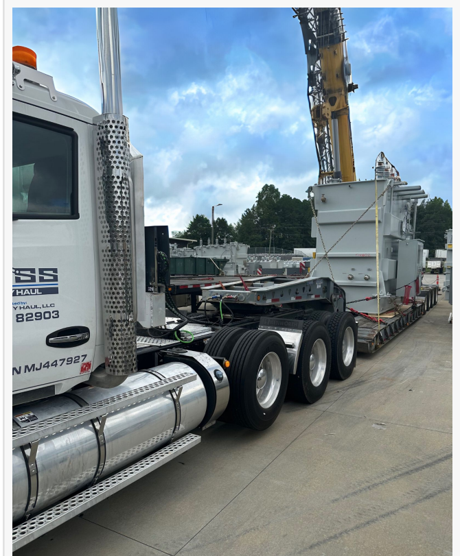
BOSS Heavy Haul recently completed its inaugural project from its new Lake City, Ga. yard, safely and efficiently transporting a 76,000-pound transformer. The team expertly hauled the load to the site, then skillfully slid and positioned it onto its foundation.
