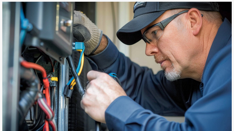
AC Repair Service in Covina
