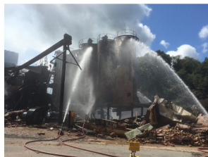
Entire facility destruction at Bosley Mill in Congleton, United Kingdom, where a fatal sawdust explosion killed four workers in July 2015 (Photos Courtesy of the Cheshire Fire and Rescue Service).
