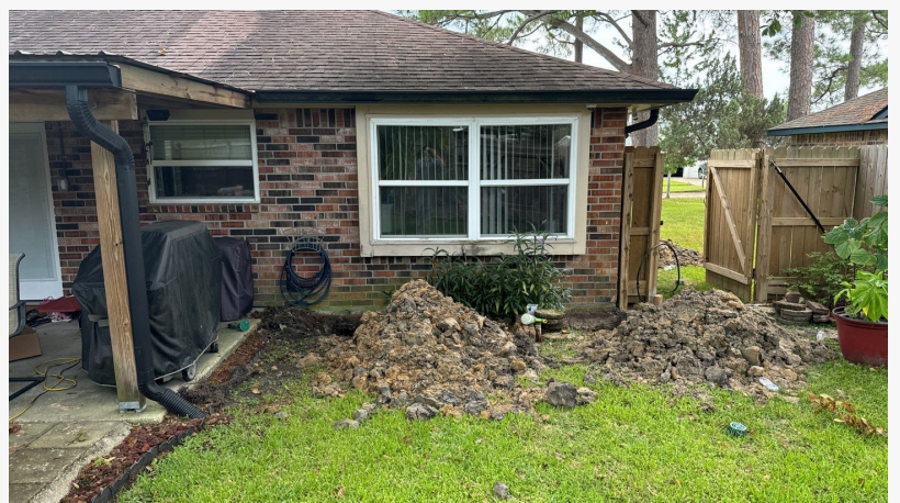
Slidell Foundation Repair
