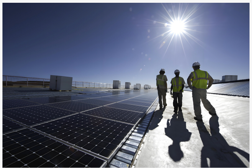
Photovoltaic panel installation
