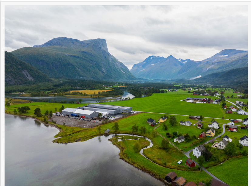
Factory and surrounding area
