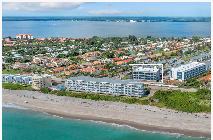
Harbor Island Beach Club, Building A | 3051 Hafen Lane, Melbourne Beach, Florida
