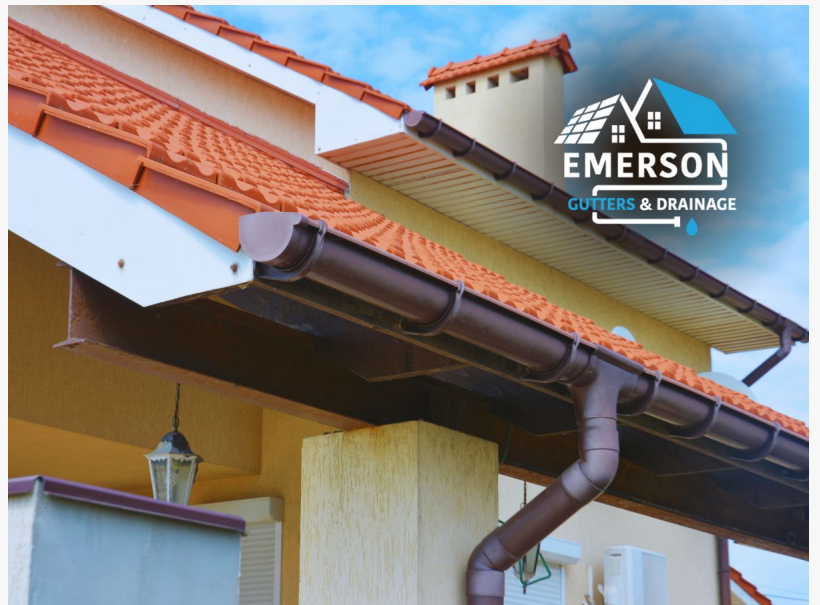
Gutters and Drainage by Emerson Pro Services
