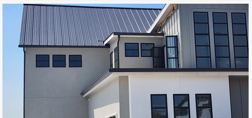
Seamless Gutter Installation by Emerson Pro Services
