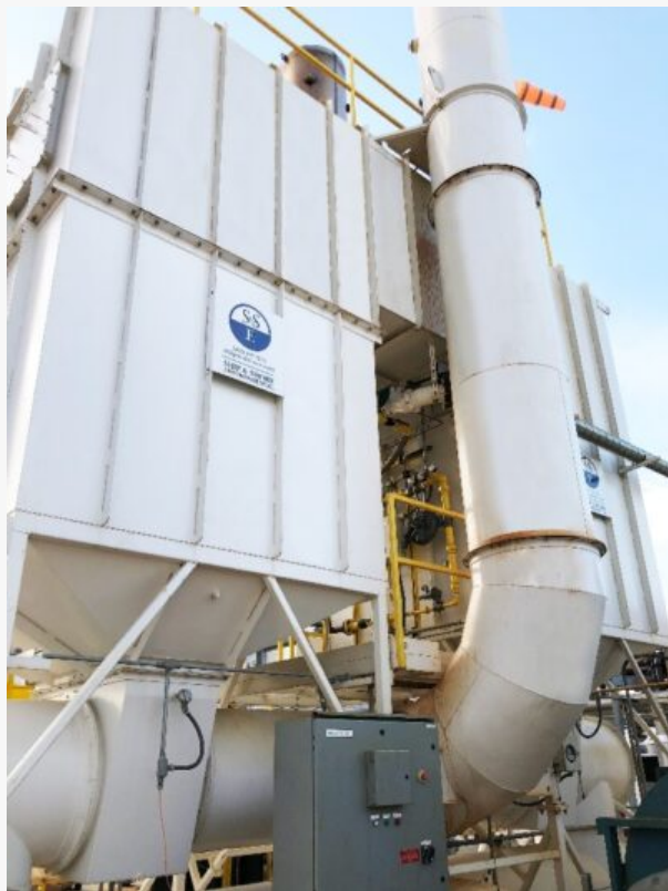
Ship & Shore 15,000 SCFM RTO for a Biogas Customer
