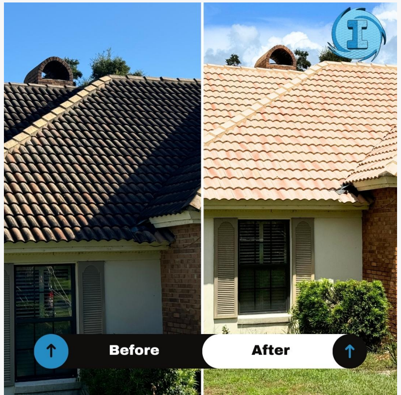
Stunning Roof Transformation in Wekiva Springs
