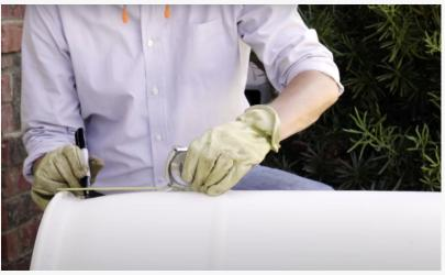
The first step of the build is to measure where the spigot and overflow holes will be drilled.
