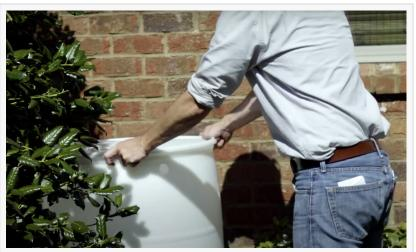
Place the completed rain barrel next to or adjacent to the downspout with the overflow pointing away from the house.
