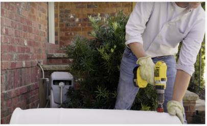
Use a drill to cut the holes for the spigot and overflow.
