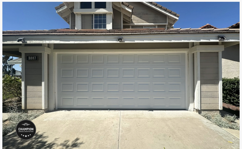
Garage Door Repair Garden Grove CA - After
