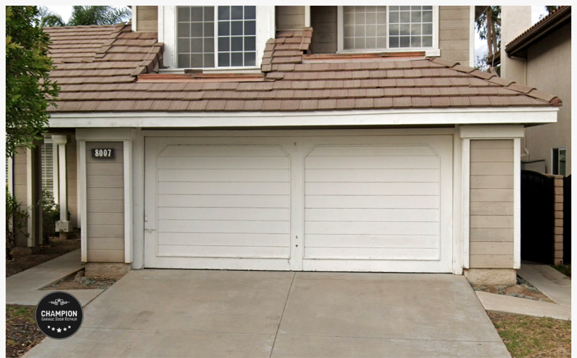
Garage Door Repair Garden Grove CA - Before
