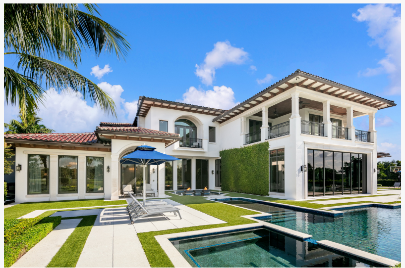
Waterfront construction Fort Lauderdale
