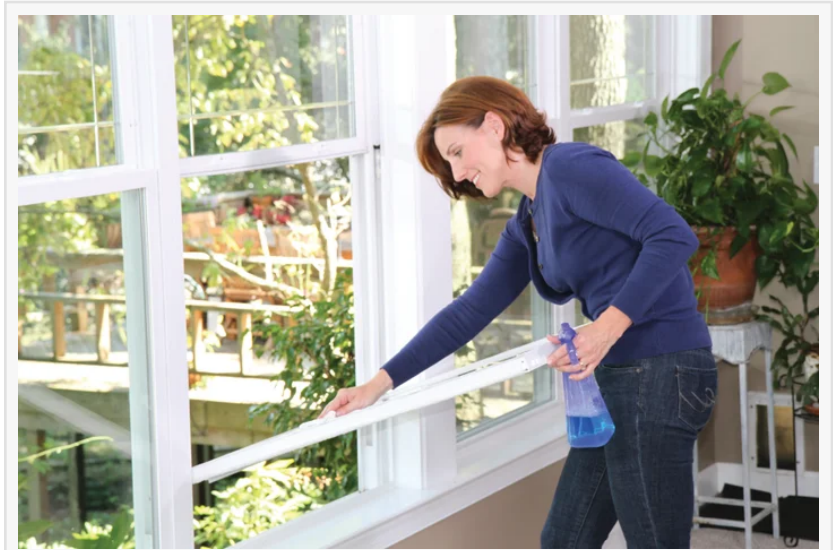
Window Sash Removal
