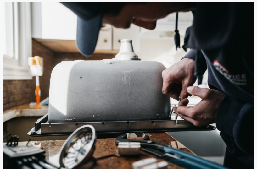
Plumbing Repair Services Saskatoon
