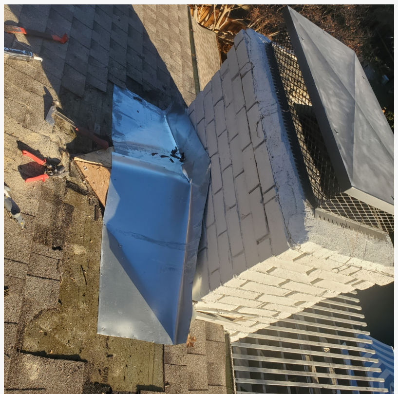
Chimney Flashing by Emerson Pro Services
