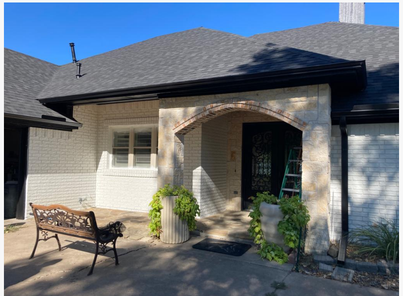
Concrete Construction by Emerson Pro Services
