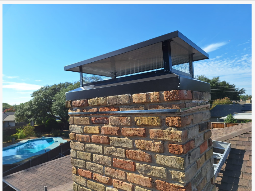
Chimney Capping by Emerson Pro Services
