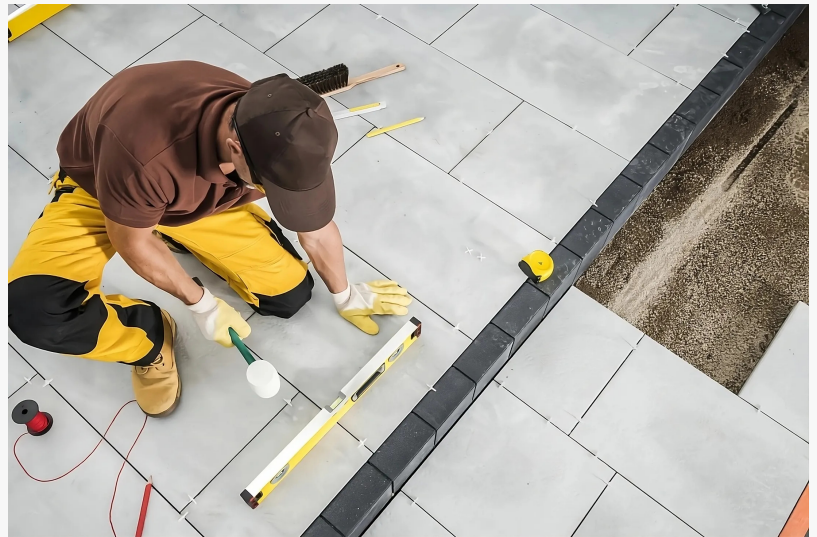
Paving Services by Emerson Pro Services
