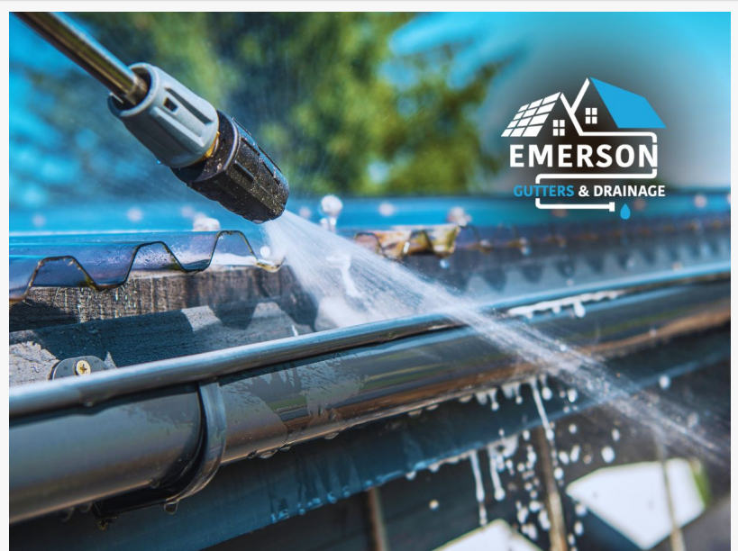
Gutter Maintenance by Emerson Pro Services
