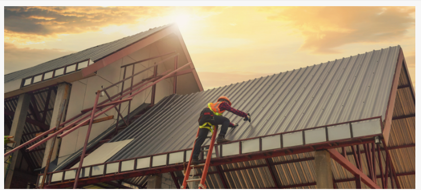
Roofing Installation Services
