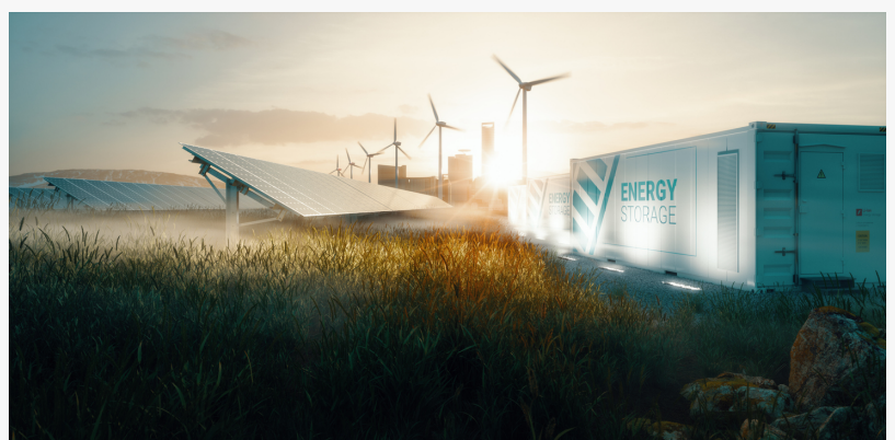
Hydrogen Energy Storage Market
