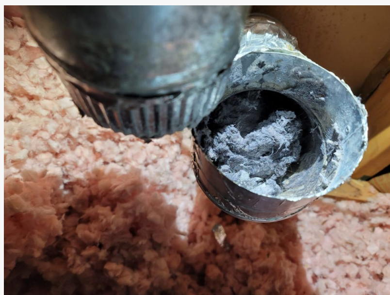
Air Duct Cleaning with Emerson Pro Services
