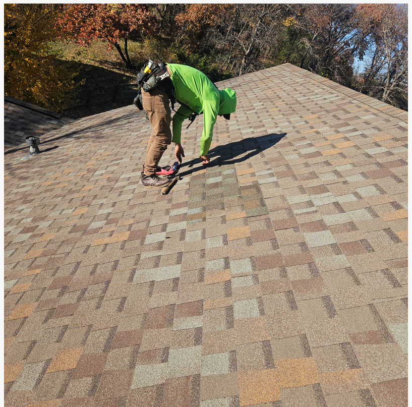
Roof Maintenance and Inspection
