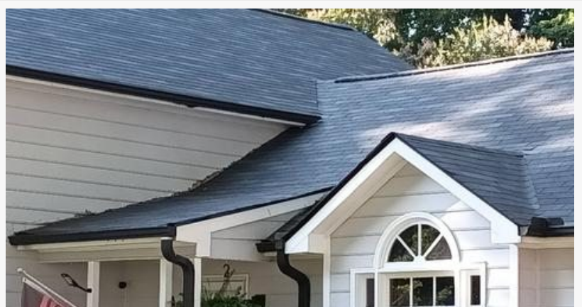
Roof Installation by Emerson Pro Services
