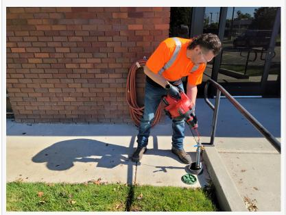
Electro Scan's SWORDFISH inspects water service lines for lead, without digging or excavation.
