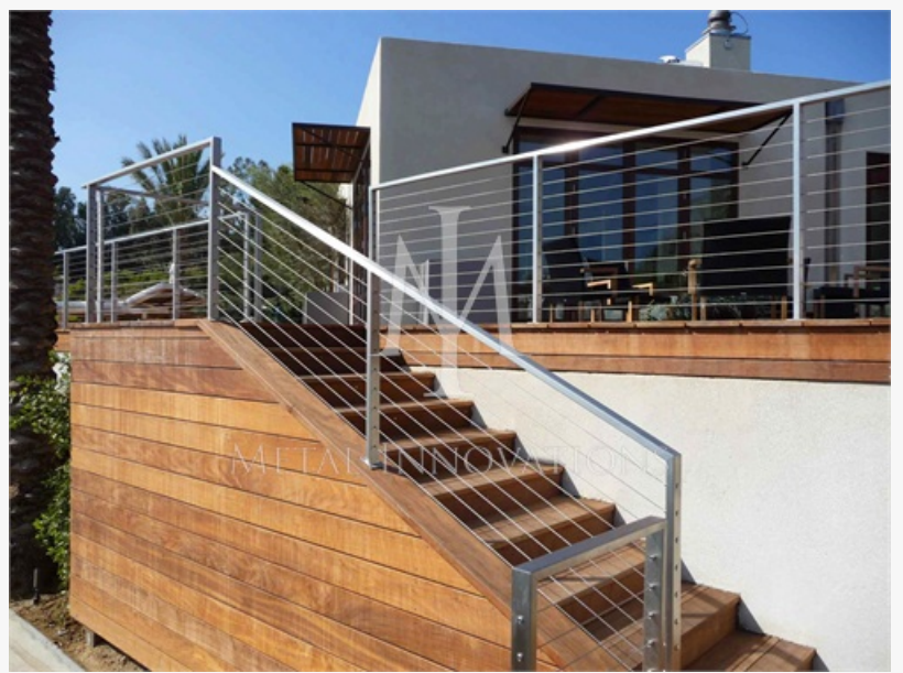
Metal Innovations Cable Railing Installation Exterior
