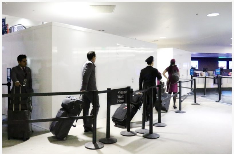
SwiftWall temporary wall systems in Los Angeles International Airport
