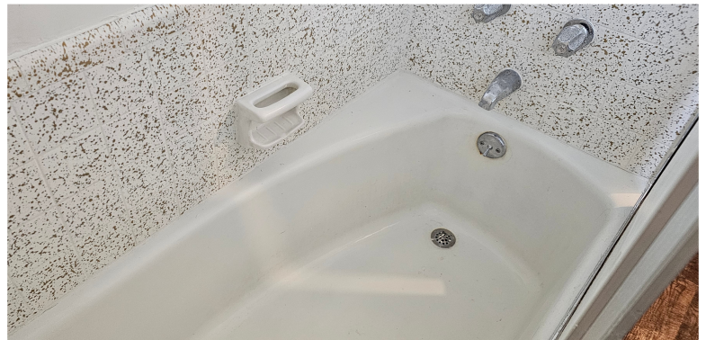
Hollywood tile restoration and regrouting
