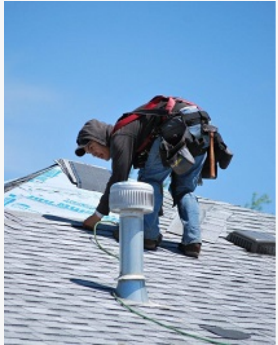
Tile roof repair Los Angeles
