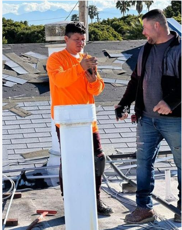
Flat roof repair Los Angeles
