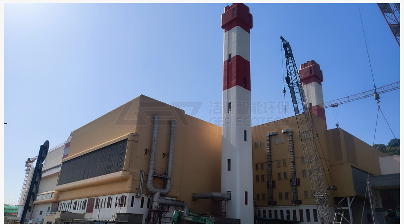
Macao Waste Incineration Plant
