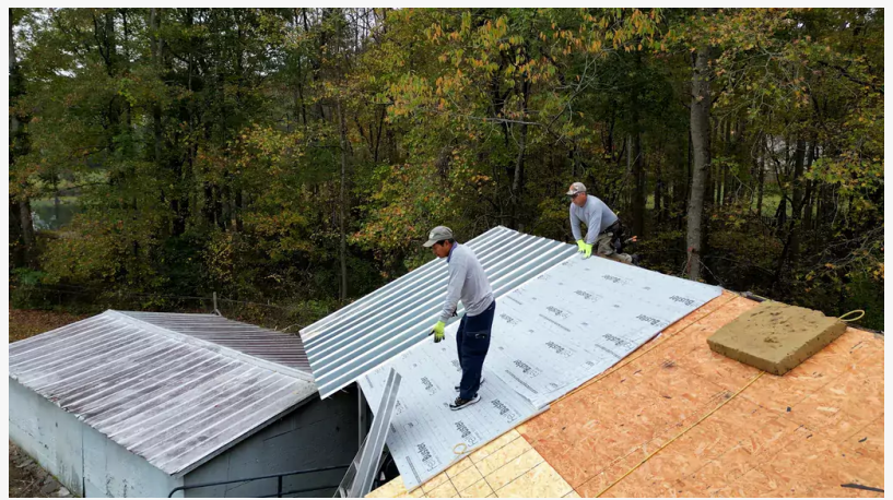
Installation of Standing Seam Metal Roof
