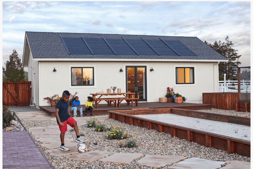
Installation of GAF Solar Shingles
