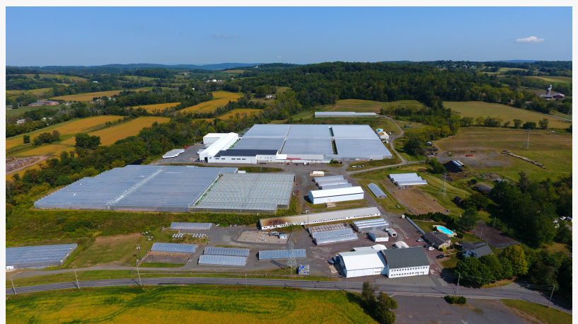
Major Greenhouse Operation
