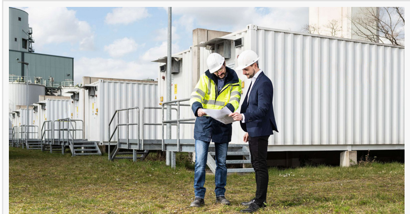
Iqony Large Scale Storage Site
